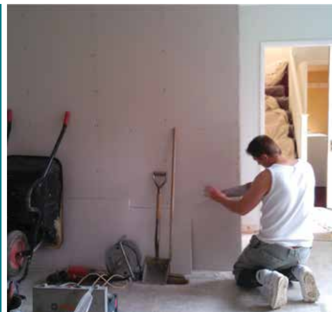
The second Norwich Hope Into Action house being refurbished
